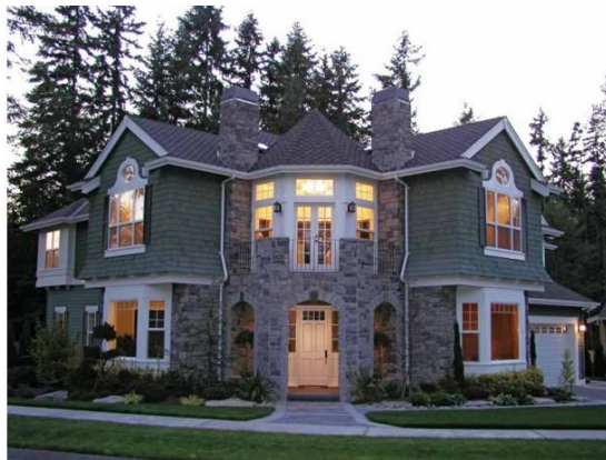
Corner unit with similar level of architectural detailing as the front elevation
