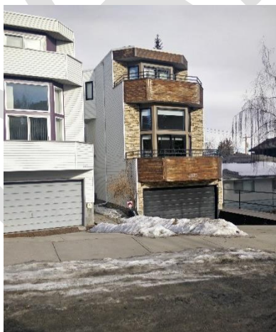
Avoid this: Inconsistent, materials or paint on side façade
