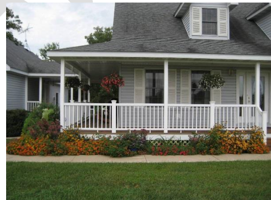
Covered front porch treatment
