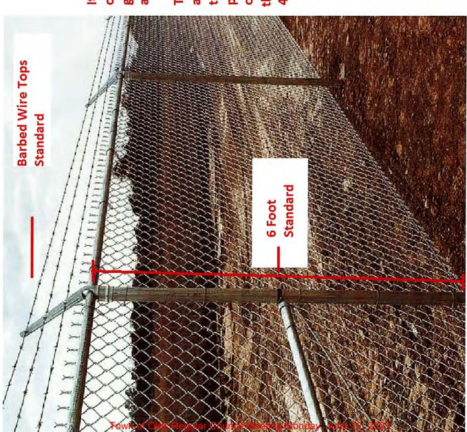
It will be a 6' standard chain link fence with galvinized steel posts and barbed wire top.
