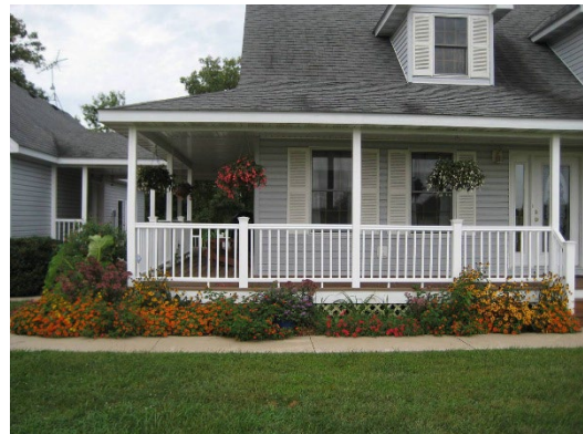
Covered front porch treatment
