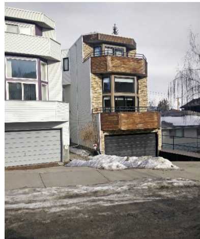
Avoid this: Inconsistent, materials or paint on side façade
