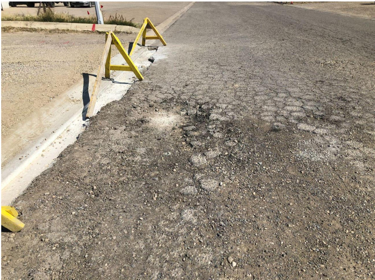
Figure 3 "Alligator Cracking"
