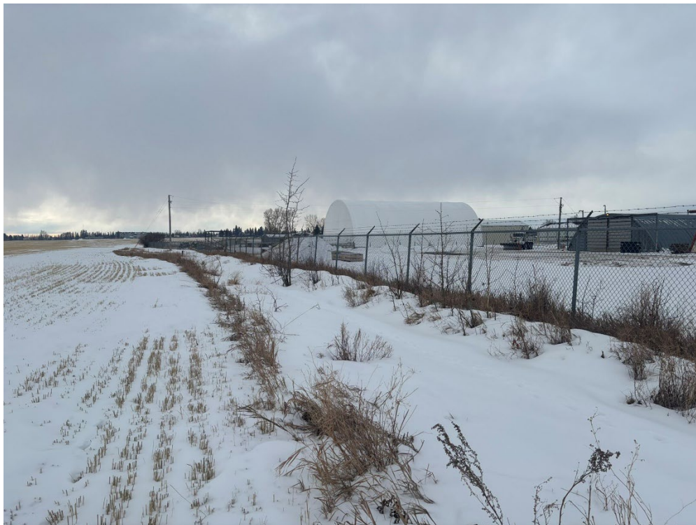
PHOTO 4. Drainage ditch on east side of highway maintenance yard, viewing south.
